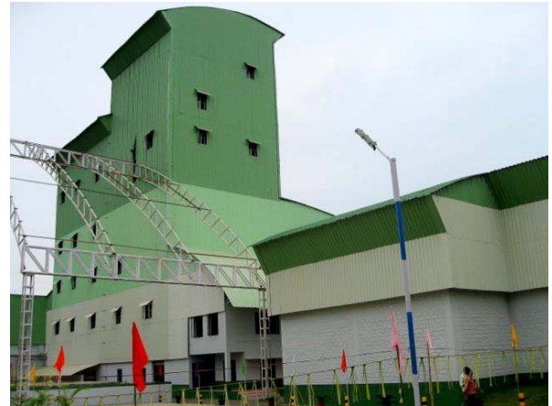
New feed mill of Kerala Solvent Extractions processing 500 tons per day.
